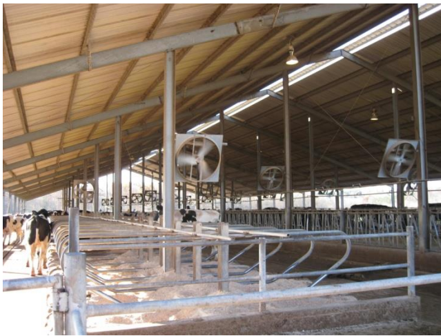
Figure 25. The ideal freestall barn maximizes natural ventilation with high, open sidewalls, a ridge vent opening and supplements natural ventilation with fans used to increase air flow and exchange.
