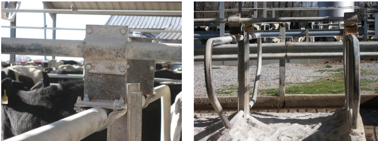
Figure 17. An example of a welded pipe fixture used to raise the height of a neck rail.
