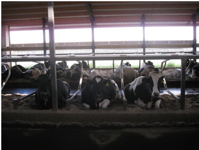
Figure 14. Lunge space can be preserved by keeping the area in front of the cows' heads free of obstructions.
