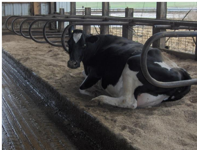
Figure 6. Detached or broken stall dividers or structures can lead to poor stall usage, dirty cows, or cow injury and entrapment.
