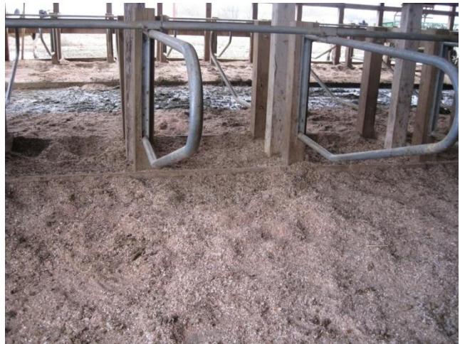
Figure 14. Lunge space can be preserved by keeping the area in front of the cows' heads free of obstructions.
